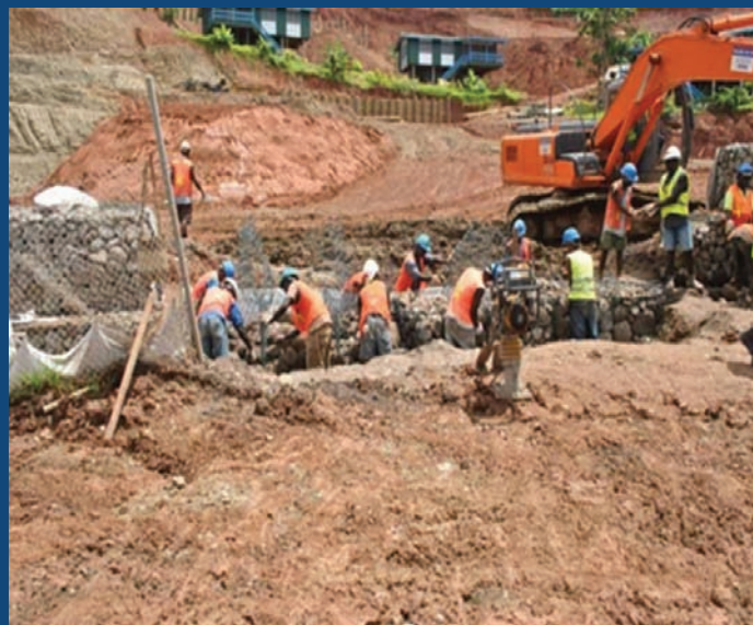
Gabion Wall Construction – Filling gap in wall
